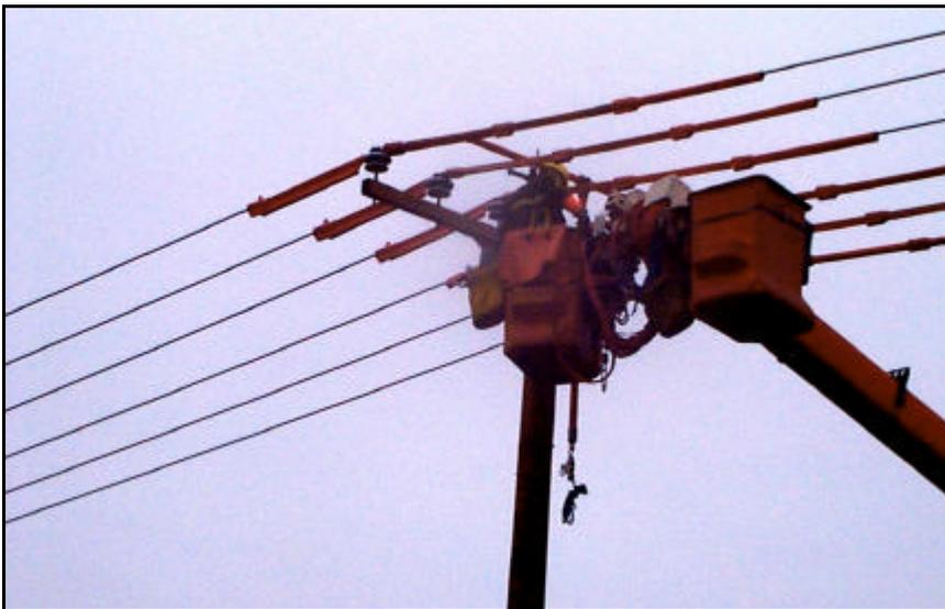
Figure 2. Gloving Method working from an Insulating Aerial Device.
