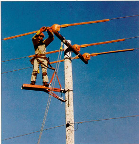
Figure 1. Gloving Method working from an Insulating Platform
