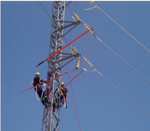
Figure 3. Stick Method working from the structure
