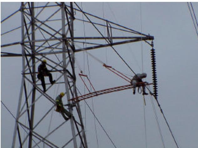
Figure 4. Barehand Method working from the insulating ladder
