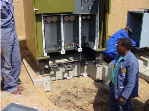
**Photo 12 – Front cable access to compact switchgear**
