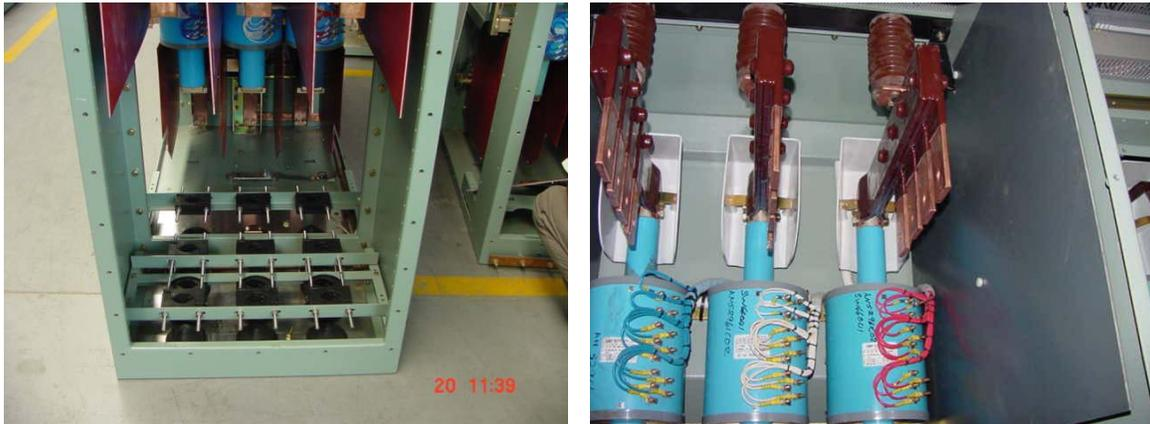
**Photo 9 – Provision for incoming cables on 2500 A panels**
