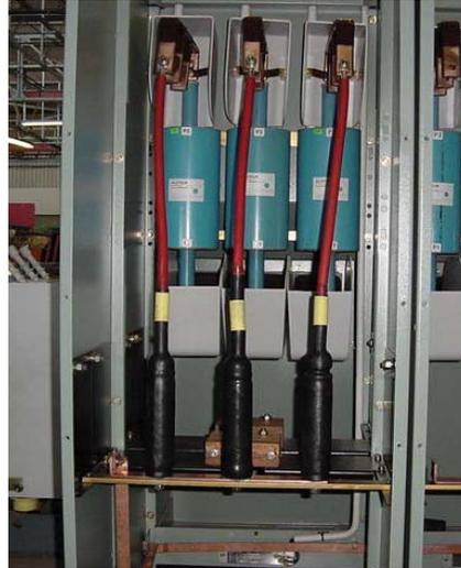
**Photo 11 – Indoor surge arresters fitted with sufficient clearances**
