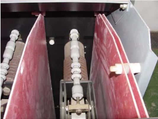
**Photo 4 – Differing specific creepages applied in switchgear**
