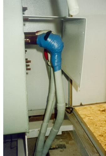
**Photo 1 – Oil-filled RMU bushing arrangement**
