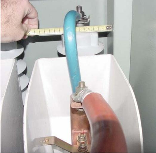
**Photo 10 – Outdoor surge arresters fitted with insufficient clearances**
