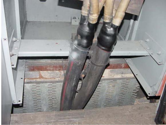
**Photo 3 – Unsupported MV cables terminated into switchgear**
