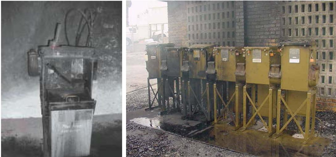
**Photo 1 – Examples of switchgear failures due to an internal arc fault in oil**
