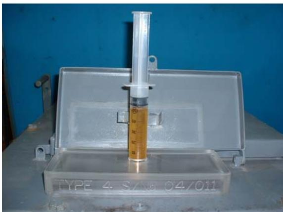
Fig. 5 Test access cover plate and sample kit fitted on a Ring Main Unit
