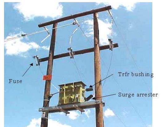
It was during this period that an effort was made within Eskom to improve on surge arrester maintenance mainly on 11kv and 22kv Distribution lines. Pole mounted transformer losses within Eskom distribution was calculated to be approximately four times higher than the average utility and this situation had to be addressed.
