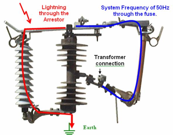
This configuration performed better under normal 50hz conditions and when exposed to over voltage occurrences such as lightning the surge arrester could now affectively deal with the over voltage occurrences. No more nuisance fuse blows or transformer losses.
