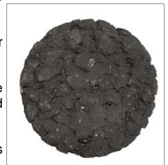
Typical core sample of a road surface
