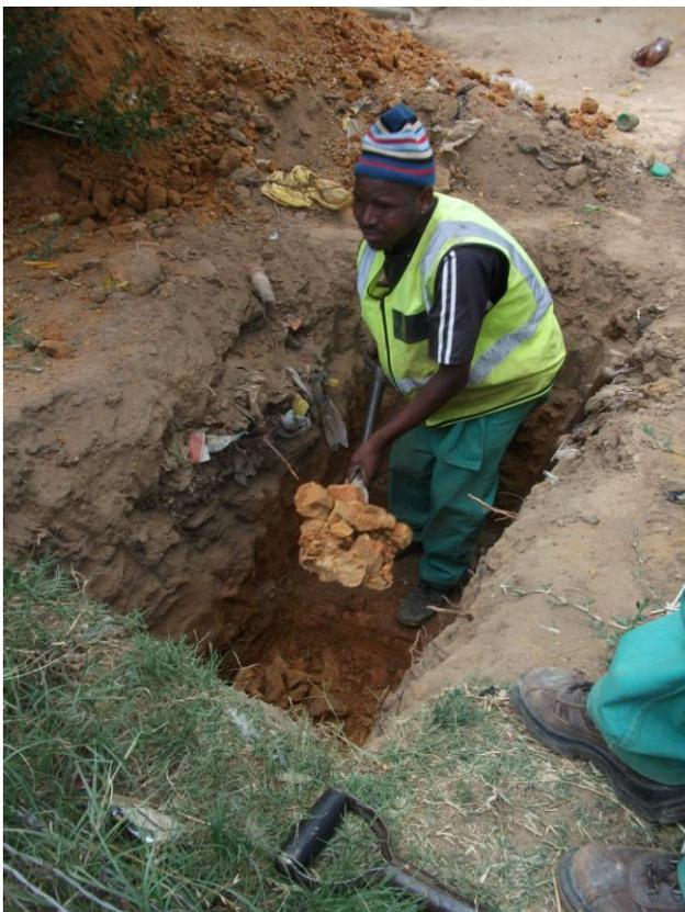
**Figure 2: The planting of an electric pole by a local labourer**
