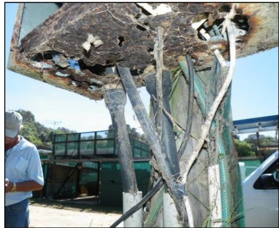
Fig. 2.3: Pictures of Unsafe Conditions of Electricity Circuitry within the Caravan Park (2)
