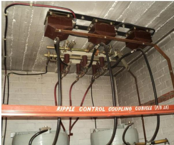
*Illustration 1 Ripple Control Coupling Cell*
