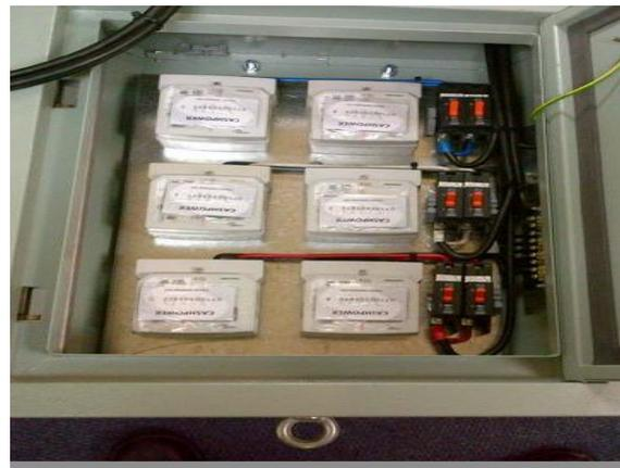
Figure 8: Protective Enclosure Unit with Meters
